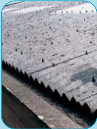
Asbestos cement roof
